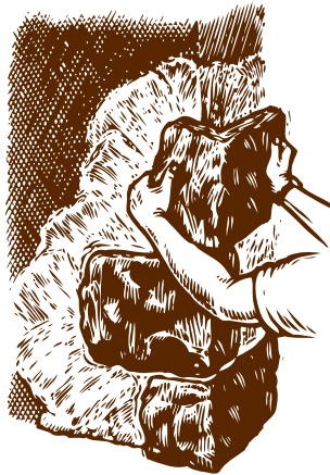
FIG. 5 Install Corners First
