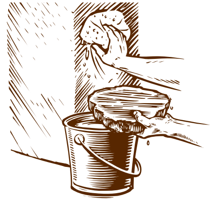
FIG. 3 Wet the Scratch Coat and Veneer
