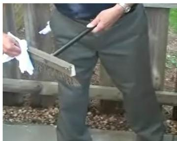
Tap the squeegee periodically to remove excess material. Using an old towel, wipe the squeegee to remove all material prior to finishing.
