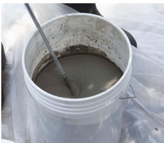
Add clean potable water and then the Flo-Coat Concrete Resurfacer into a 5-gallon pail.
