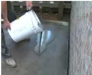
Pour the mixed product onto the properly prepped concrete surface.
