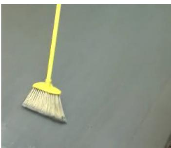
Once the product has been applied smoothly and evenly over the entire surface, take a broom and add texture to the surface. This is to prevent the concrete from being slick when finished.
