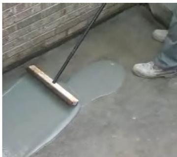
Using a squeegee, pull the material across the concrete surface to spread it evenly. Flo-Coat Resurfacer may be applied from feather edge to 1/2" in thickness.
